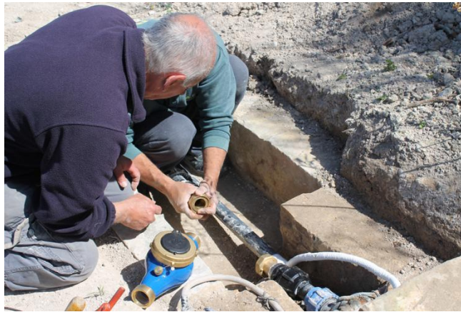
Figure 7.3: Flow meter being fitted to an agricultural groundwater abstraction source
