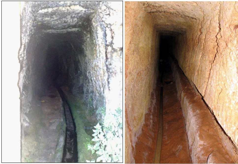
Figure 5.18: Typical spring channels in the perched aquifer system, showing the nature of groundwater flow in these aquifer systems, and the difficulties associated with the installation of water level and water flow monitoring instrumentation
