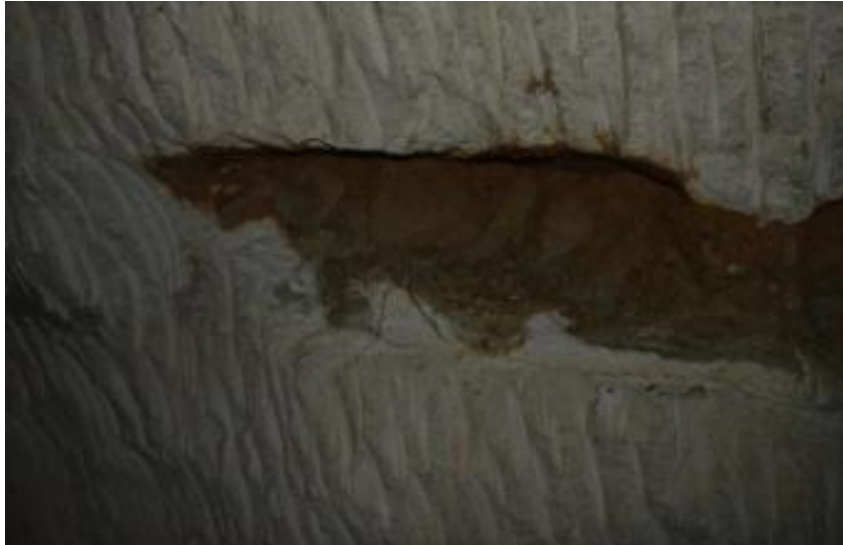
Figure 2.54: Weathered horizontal discontinuities with fine clay infill, resulting from dissolution in the LCL
